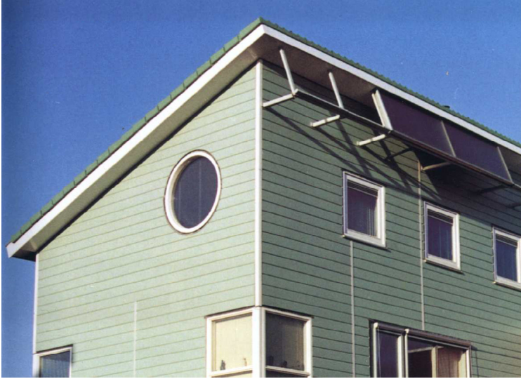
Figure 13: This north-facing roof was not suitable for integration so the architect used the south facade in a creative way.
