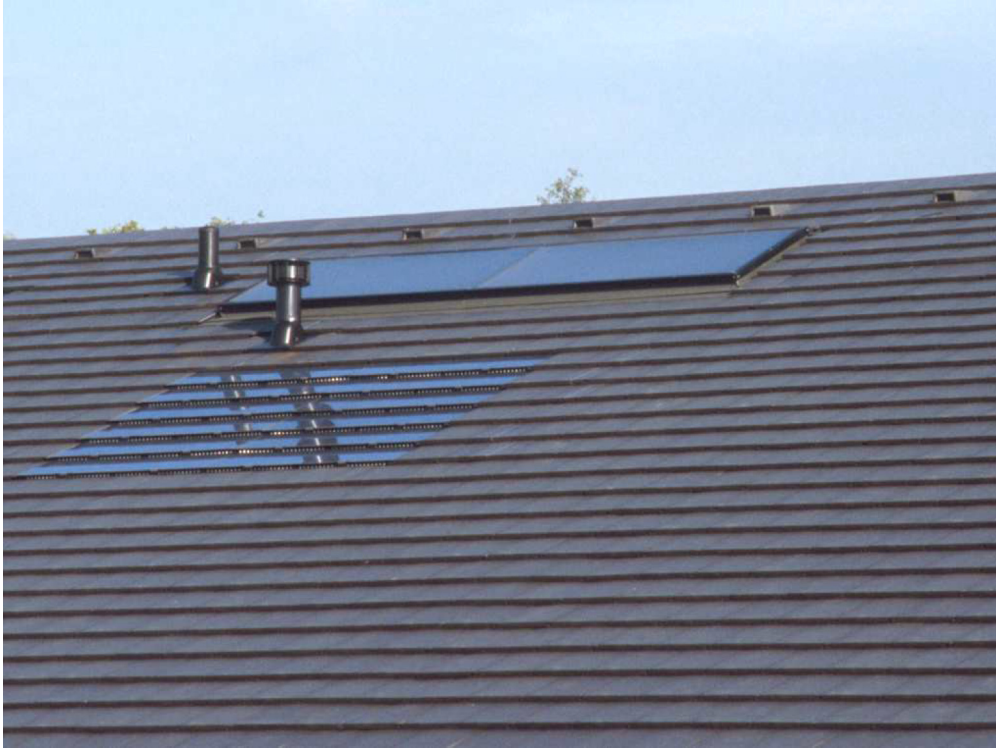
Figure 11: Small domestic hot water system
