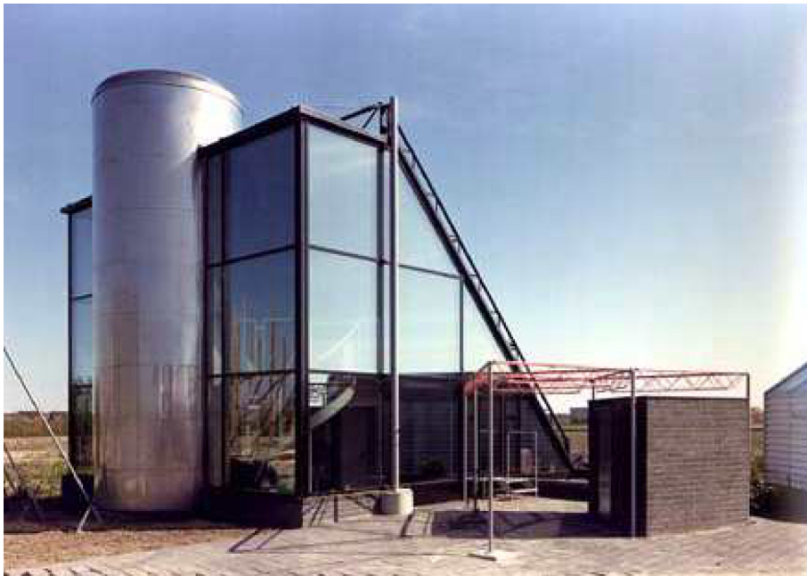
Figure 17: This house uses a huge 40 m 3 storage tank for a thermal solar heating system for space heating and domestic hot water use.
