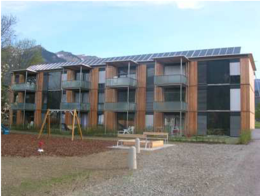
Figure 9: Example of a solar water heater for a multifamily house (Source: AKS DOMA)
