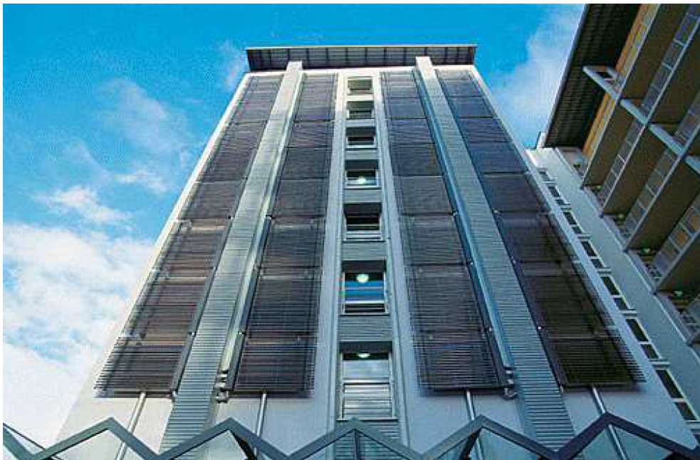
Figure 20: Student apartment block in Germany, the façade is covered with evacuated solar tubes.
