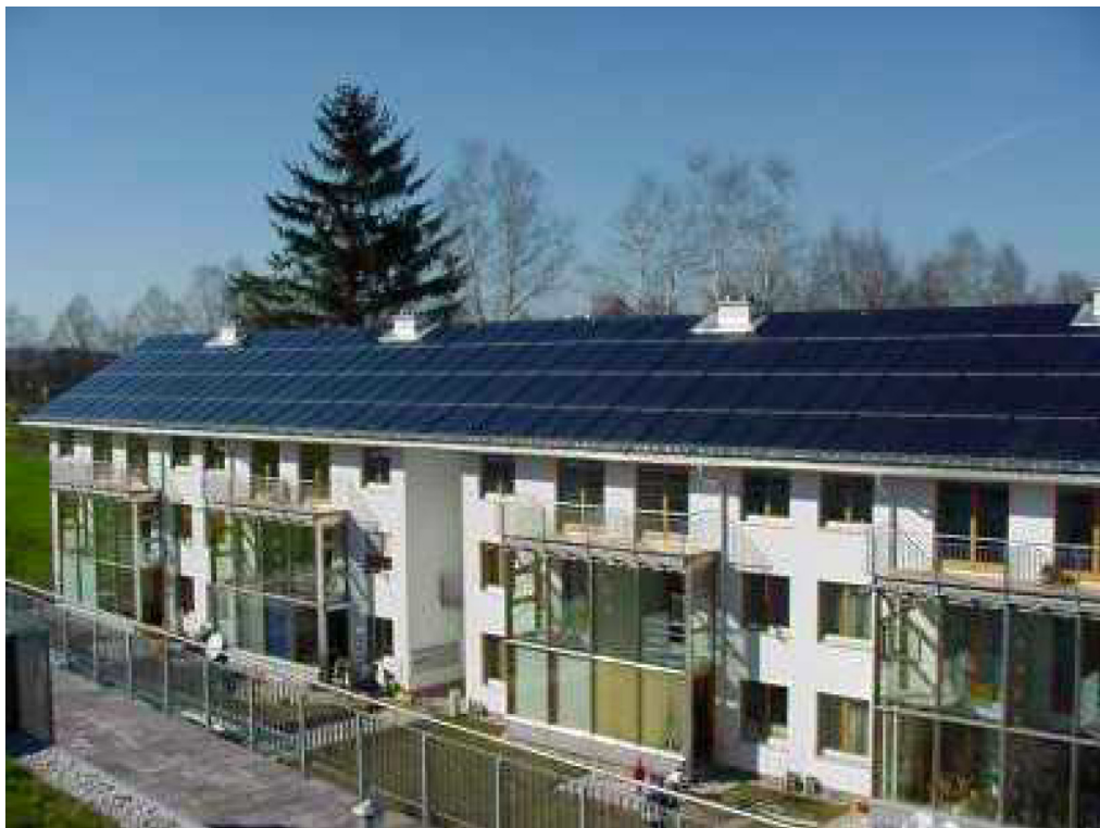
Figure 12: The fully integrated solar roof. This solution is suitable for smaller apartment buildings.
