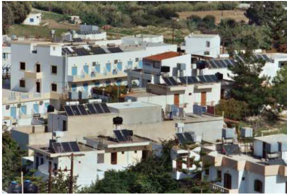
Figure 4: Thermosiphon systems in Greece
